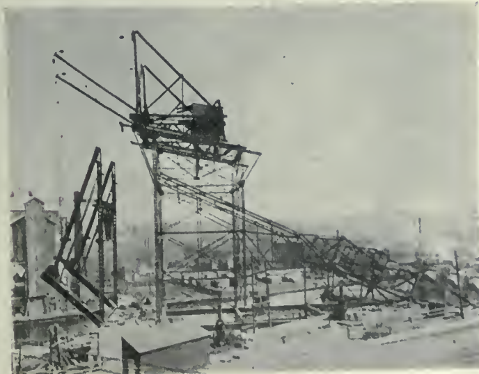
Fig. 1—Traveller on Steel Tower erecting end panel of Arch
